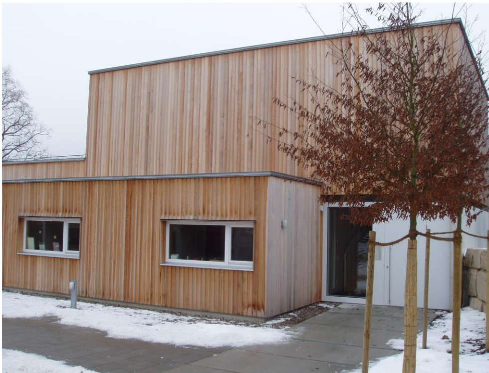
Figure 4. Holy Family Nursery in Eichstätt (Germany), designed by architect Karl Frey: cross-laminated timber panels solve vertical and horizontal structural elements.
