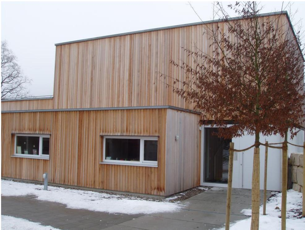
Figure 4. Holy Family Nursery in Eichstätt (Germany), designed by architect Karl Frey: cross-laminated timber panels solve vertical and horizontal structural elements.
