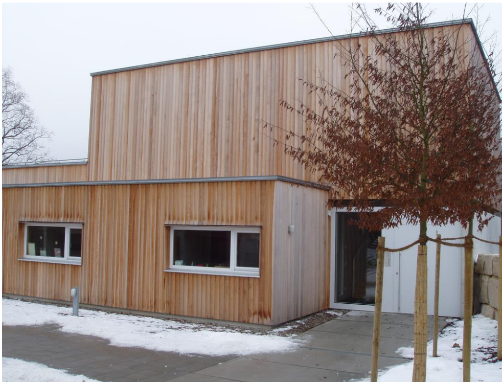
Figure 4. Holy Family Nursery in Eichstätt (Germany), designed by architect Karl Frey: cross-laminated timber panels solve vertical and horizontal structural elements.
