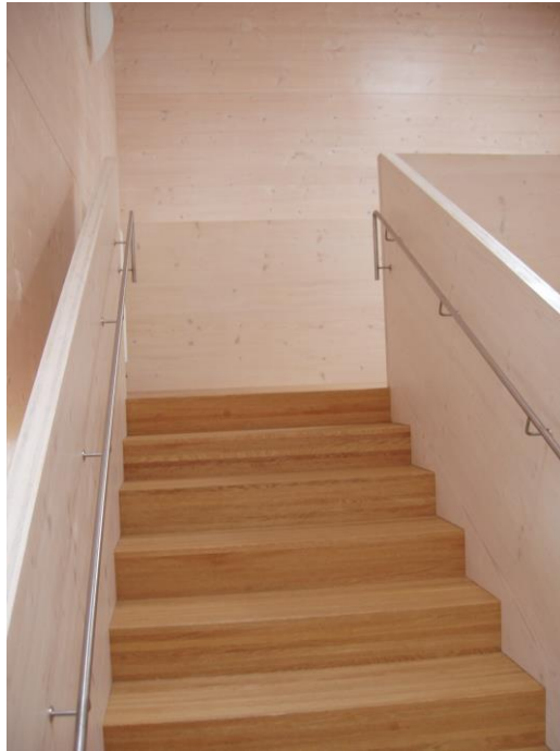
Figure 5. Holy Family Nursery in Eichstätt: structural timber panels used with an exposed surface.
