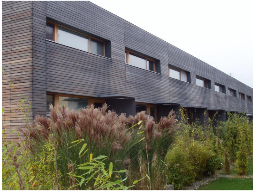
Figure 6. Passive-Energy housing in Dornbirn (Austria), designed by architect Johannes Kaufmann: the optimised section prefabricated timber panels integrate wall openings.
