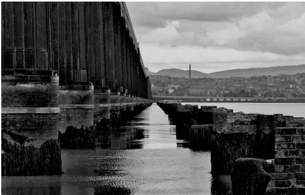
(Fig 1. Ghost Bridge/Replacement Bridge Photograph by Own Fraser McLaughlin).
